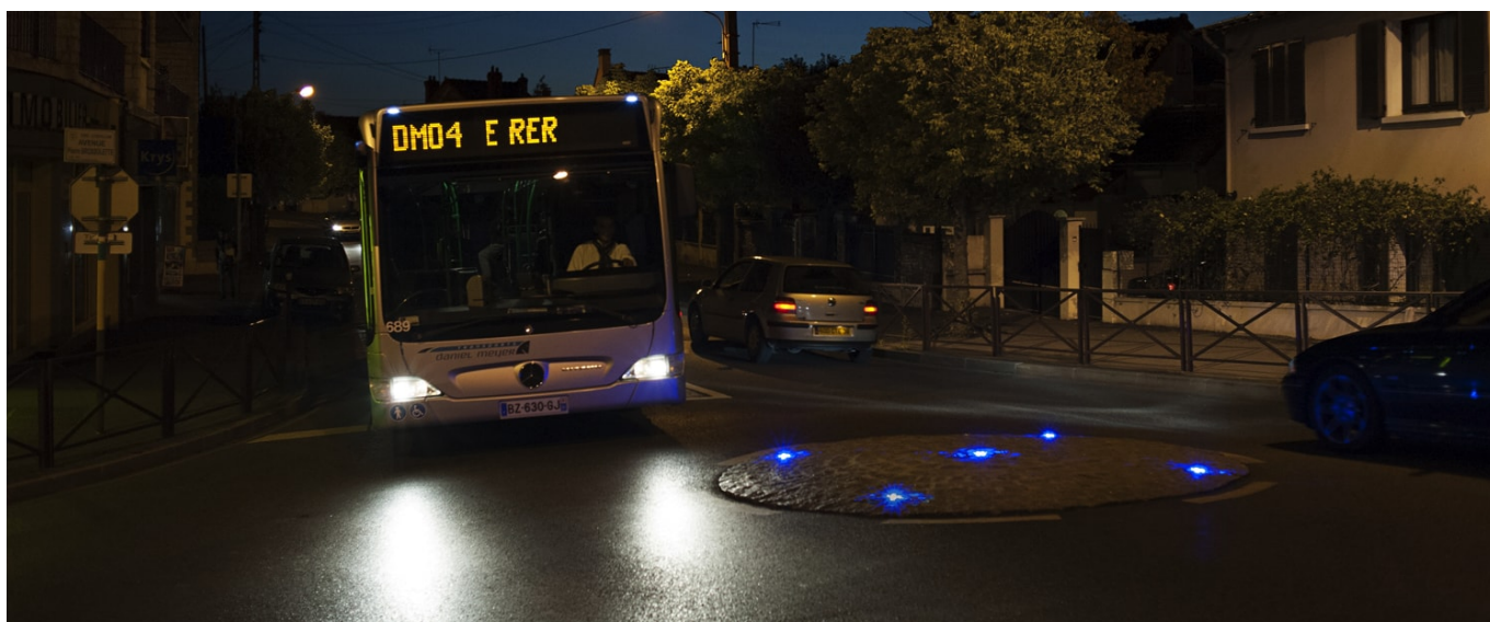
Mini-roundabout. Security marking on a vehicle-proof mini-roundabout in the city centre of Viry-Châtillon. Extra-low voltage embedded road beacon ECO-870 (constant markup with 24 blue LED visible through 360 degrees). Photography : Karolina Samborska.
