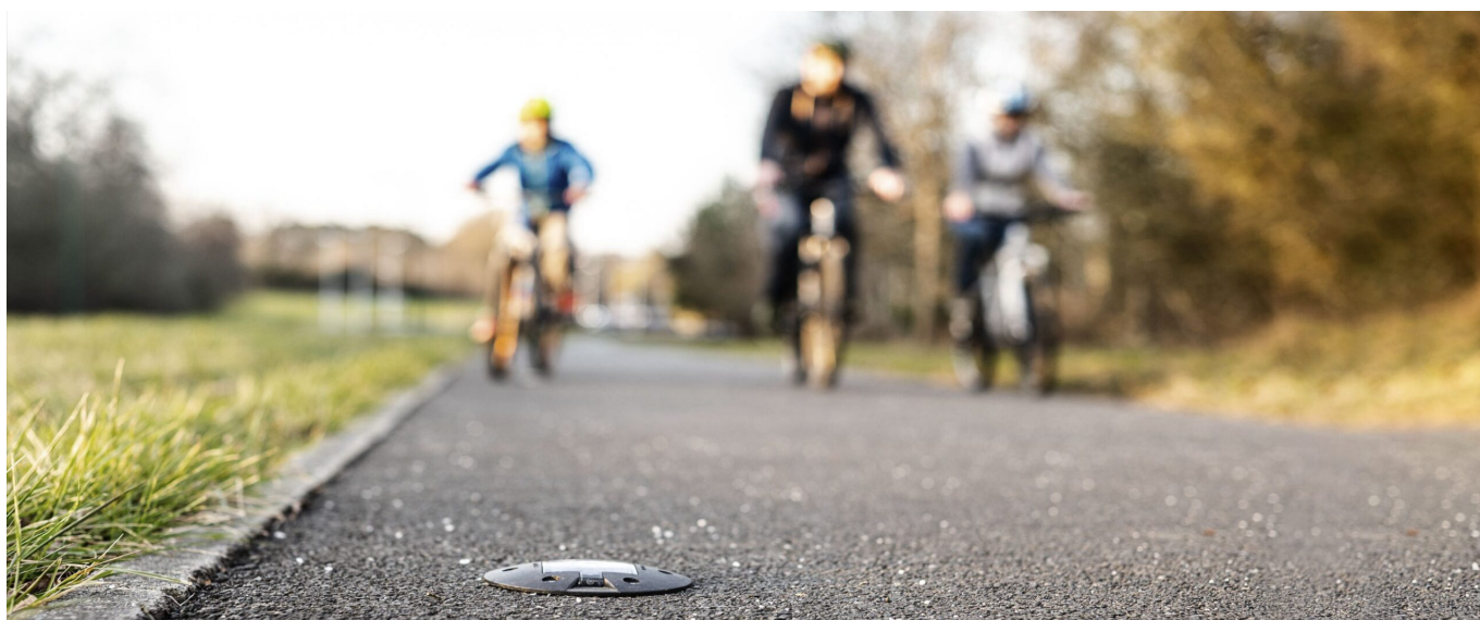
LED beaconing for a cycle path: La Vélodyssée. LED beaconing for a cycle path: La Vélodyssée. PM: Nantes Métropole, Photography: Camille Saada.
